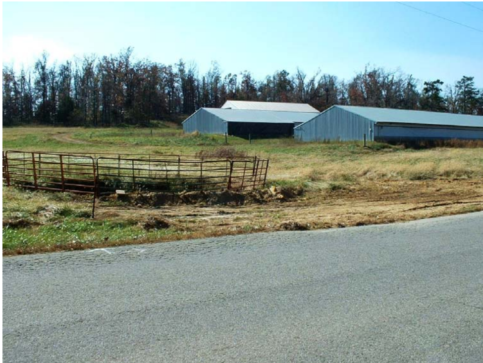
Ditch alteration and fence removal next to sinkhole. Note drainage direction sloping towards sinkhole, small berm, and fencing at edge of sinkhole. Looking southwest.
