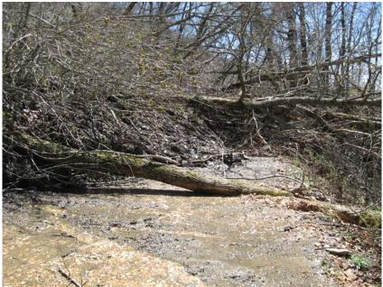
View (north side) of landslide covering road. Notice water flowing from slide onto road.
