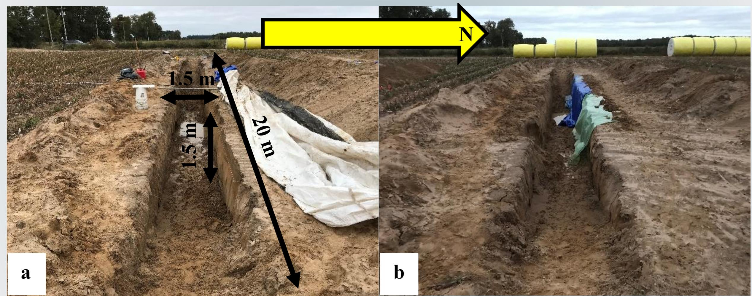
Photographs showing the trenches that were excavated at DBNW3: a) The southern trench (DBNW3S), and b) The northern trench (DBNW3N). The photographs point to the west.
