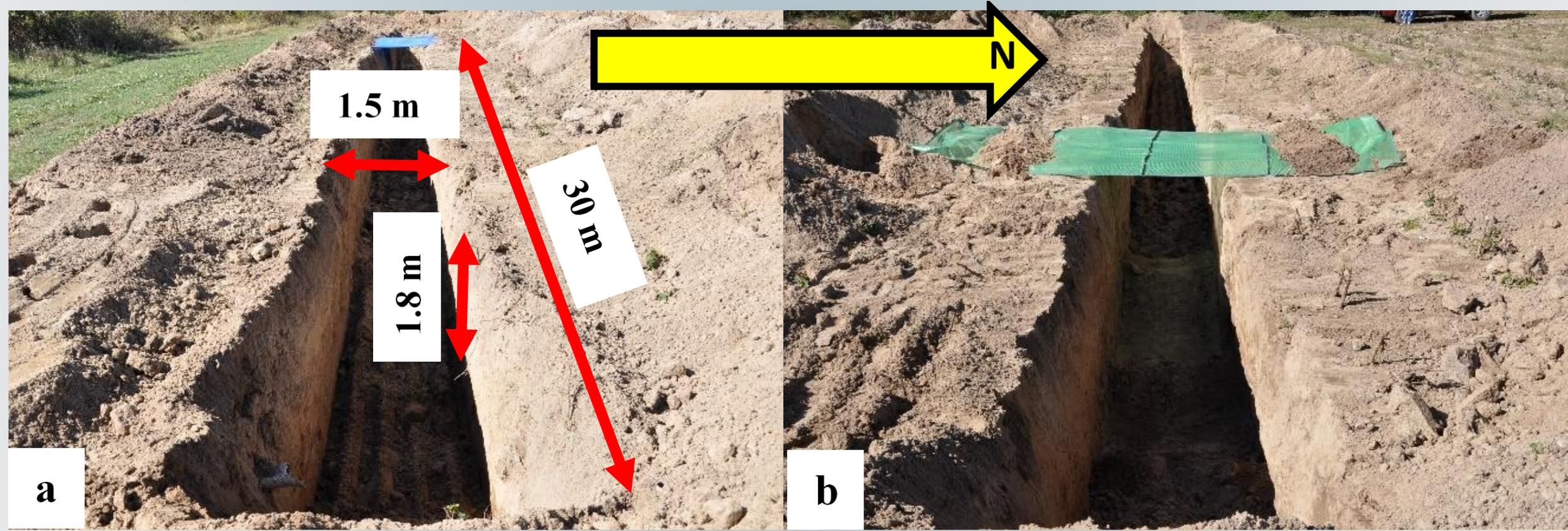
Photographs showing the trenches that were excavated at DBNW5: a) The southern trench (DBNW5S), and b) The northern trench (DBNW5N).
