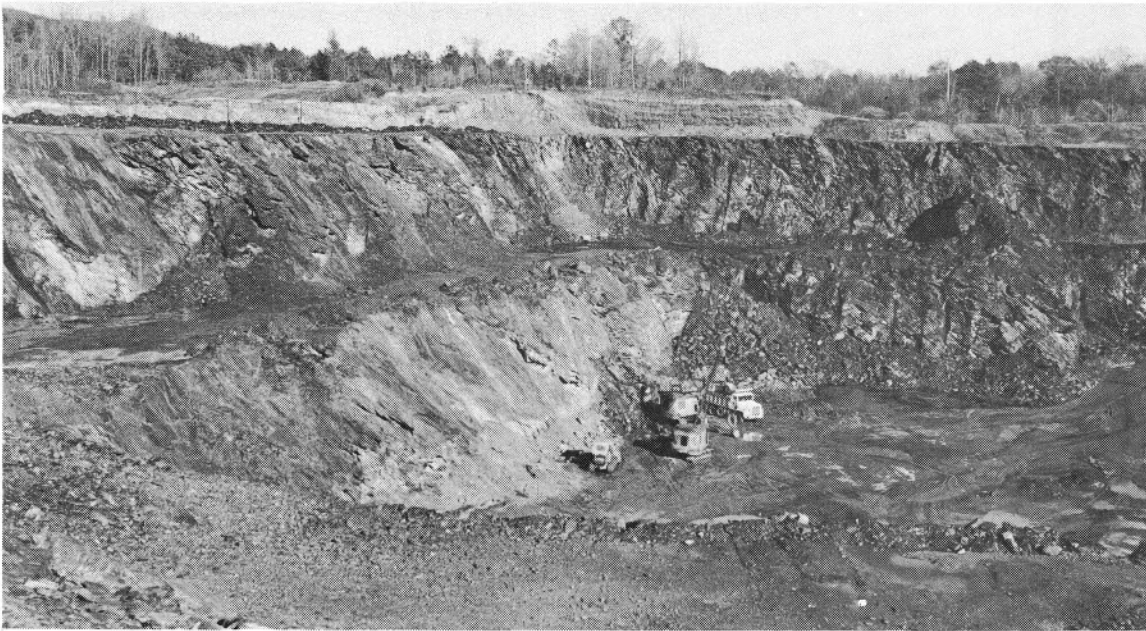
Figure 20. — Stop 15. A view of the Genstar Co. slate granule pit north of Glenwood. Sheared and faulted shale with some siltstone, graywacke, and chert in the middle part of the lower Stanley Shale.
