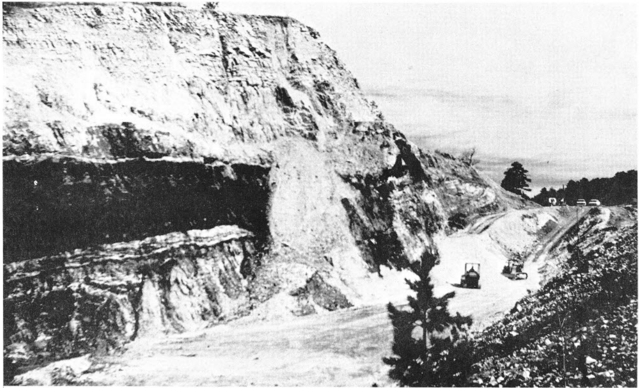
Figure 31. - Open-pit, tripoli ("Novacite®") mine of the Malvern Minerals Company, Garland County, Arkansas. The stratigraphic section is inverted here; the white, tripolitic upper member of the Arkansas Novaculite is at the base of the deposit, the dense novaculite of the lower member is at the top, and the dark shale of the middle member is between them.
