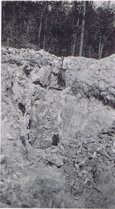
PLATE 19. Opening in sandstone on Arkansas Cinnabar Mining Company property in sec. 2, T. 7 S., R. 25 W.
