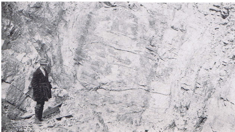
PLATE 36. View of cut across strike of sandstone and shale beds on Southwestern Quicksilver Company property in sec. 1, T. 7 S., R. 26 W. Cinnabar occurs as crystals in quartz veins. Free quicksilver also occurs here.
