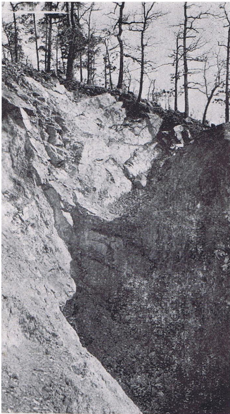
PLATE 32. View of Cut 1 on Southwestern Quicksilver Company property in sec. 6, T. 7 S., R. 25 W., showing 90 degree bend of sandstone beds.
