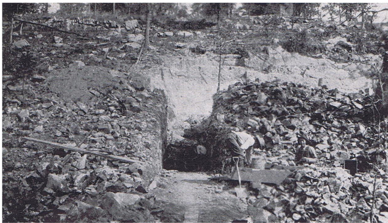
PLATE 34. View of small opening near Cut 12 on Southwestern Quicksilver Company property in sec. 6, T. 7 S., R. 25 W., showing hand sorting in cut and resorting at mouth of cut.
