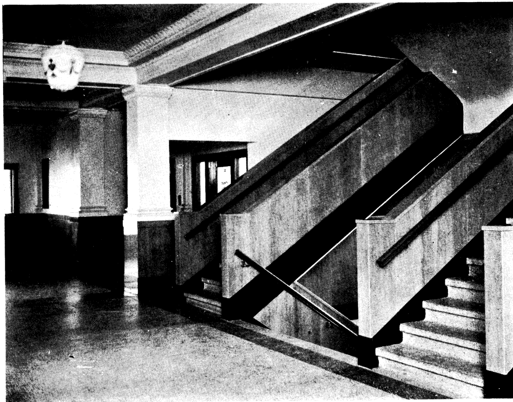
B. Arkansas black marble installation in Lincoln County Courthouse, North Platte, Nebraska.
