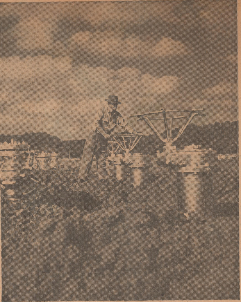
A crew of welders (left) completes the last stretch of mileage for a 30-inch natural gas pipeline in central Arkansas by joining a crossing under a highway near Little Rock. New valve installations (right) set inland from the east bank of the Mississippi River mark the point where three heavy river crossing lines merge with the main 30-inch Texas Illinois line.
