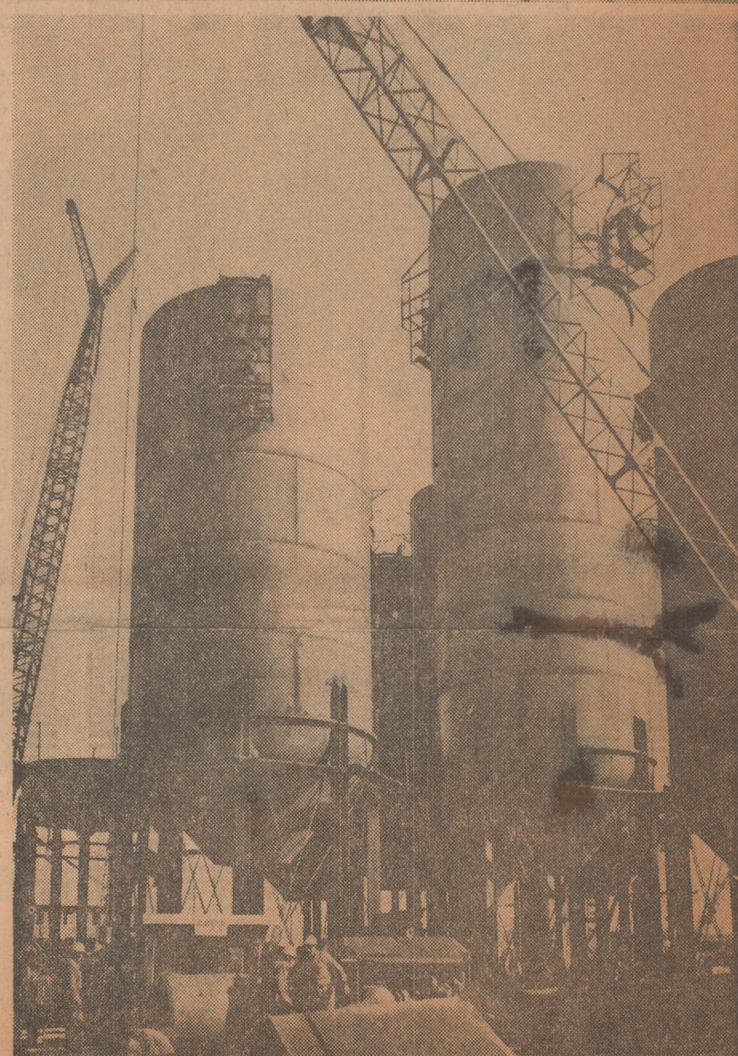
The big battery of tanks at the Alcoa plant will hold 150,000 gallons of liquid each.
