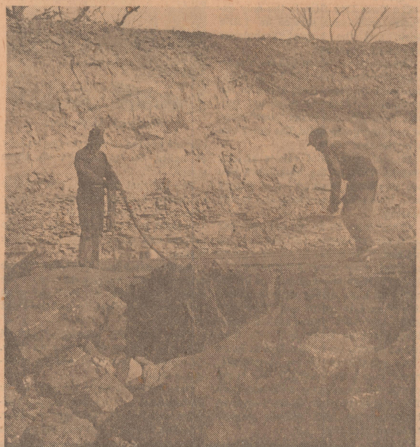
After the blast has loosened chunks of coal from the shelf, a crew readies another series of holes for more dynamite.
