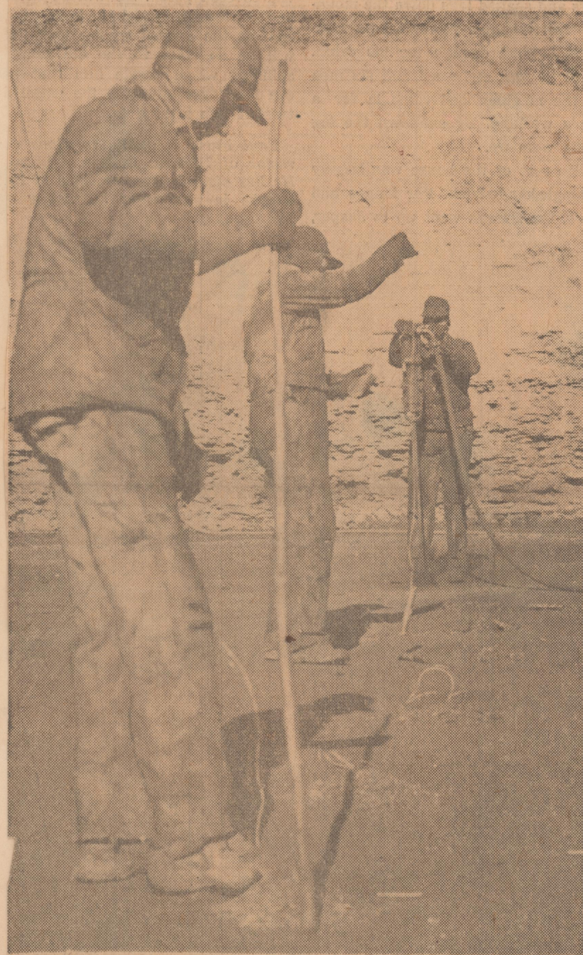
The blasting operation is reduced almost to a continuous assembly-line procedure, with the man at the jackhammer boring the holes in the coal shelf, the middle man dropping in the dynamite, and the third man tamping it in place.
