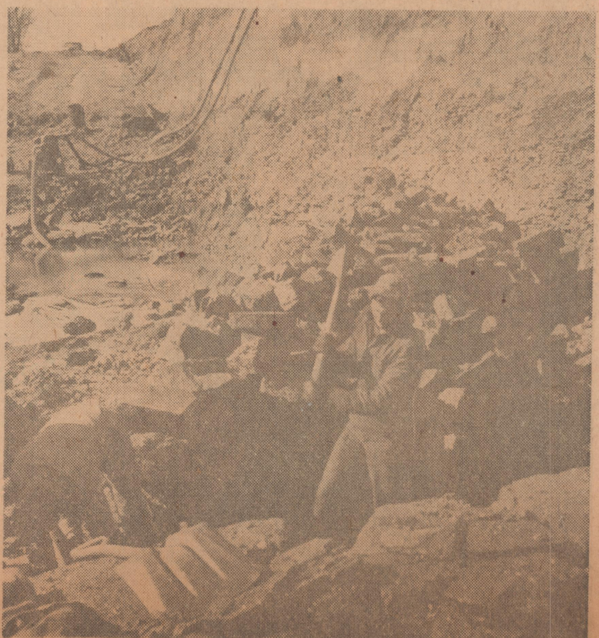
Out-size 'boulders' of coal are whacked with a sledge hammer to make for somewhat easier handling by the metal scoop of power loading equipment.
