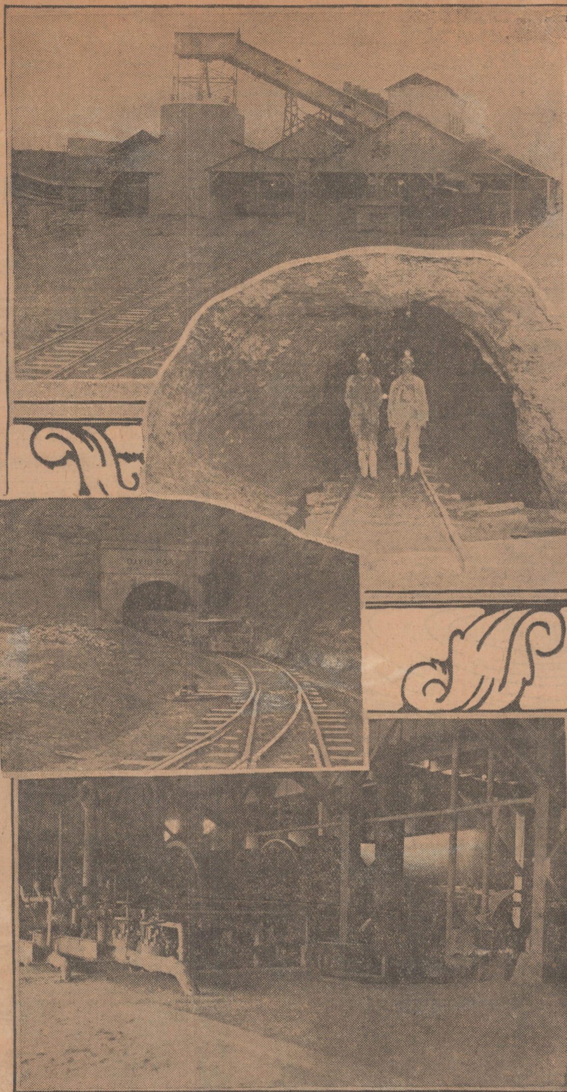
Views of the bauxite mining properties of the American Bauxite Company, in Saline county. At the top is shown one end of the big mill where the bauxite, or aluminum ore, is crushed, brought up the grade, dried and loaded in specially constructed cars for shipment to the reduction plant of the Aluminum Company of America, in East St. Louis. Immediately below the mill and at the right, is a flashlight picture taken in one of the underground workings. The walls and ceiling of this tunnel are of bauxite. At the left in the center is Davis Portal, one of the entrances to the underground mines, with a train, drawn by an electric locomotive, just emerging from the tunnel. Below is an interior view of the mill, showing a part of one of the huge rotary kilns in which the powdered ore is dried. There are a dozen of these kilns.
