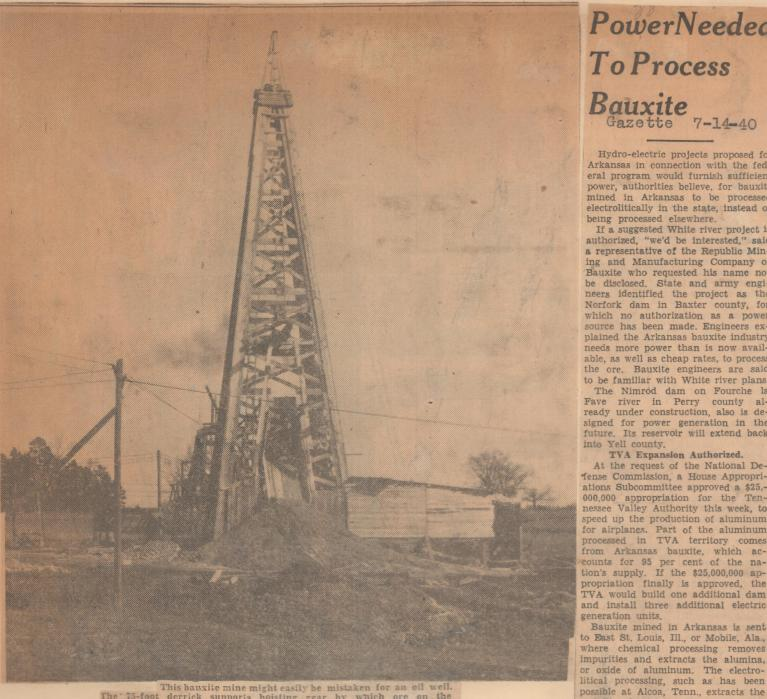
This bauxite mine might easily be mistaken for an oil well. The 75-foot derrick supports hoisting gear by which ore on the Crouch Mining Company's property south of Bauxite is brought to the surface from the tunnel 300 feet below. The company plans additional development on the 40 acres which it owns and has worked for the first time since January 1. Below the derrick a 76-inch shaft
