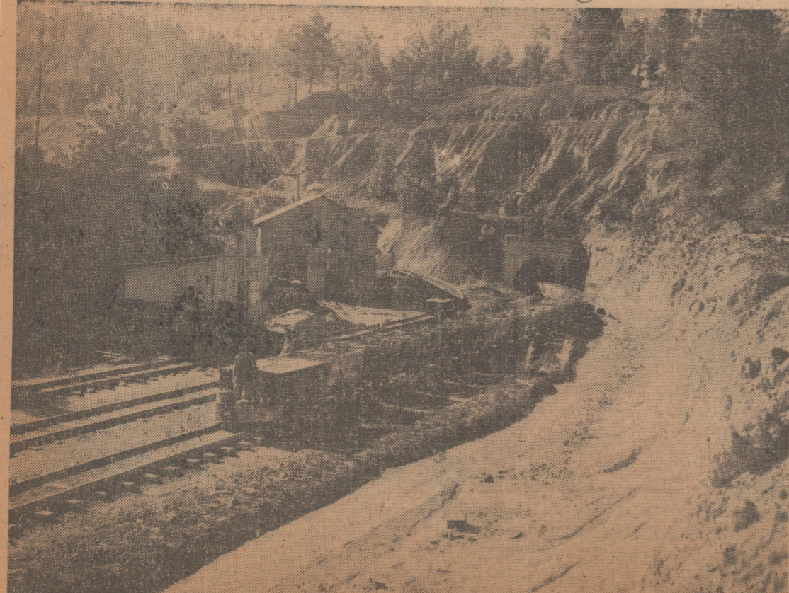
Here is the entrance of an underground Bauxite mine with a string of loaded cars being pulled to the surface by an electric mine locomotive.
