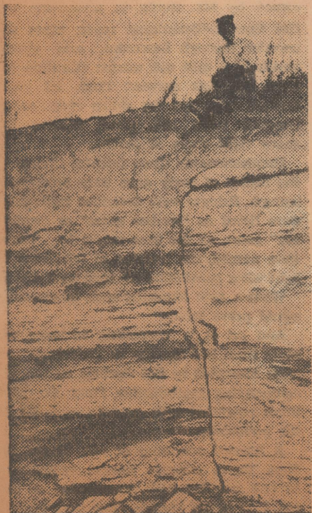
Looking at a fault in the side of a cliff.
