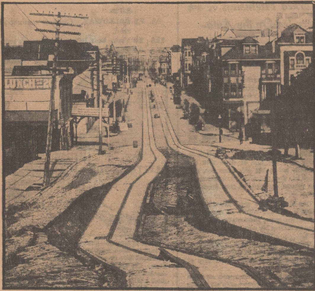
These cable-car tracks in San Francisco ran athwart the famous San Andreas fault, which slipped sideways in the classic earthquake of 1906.
