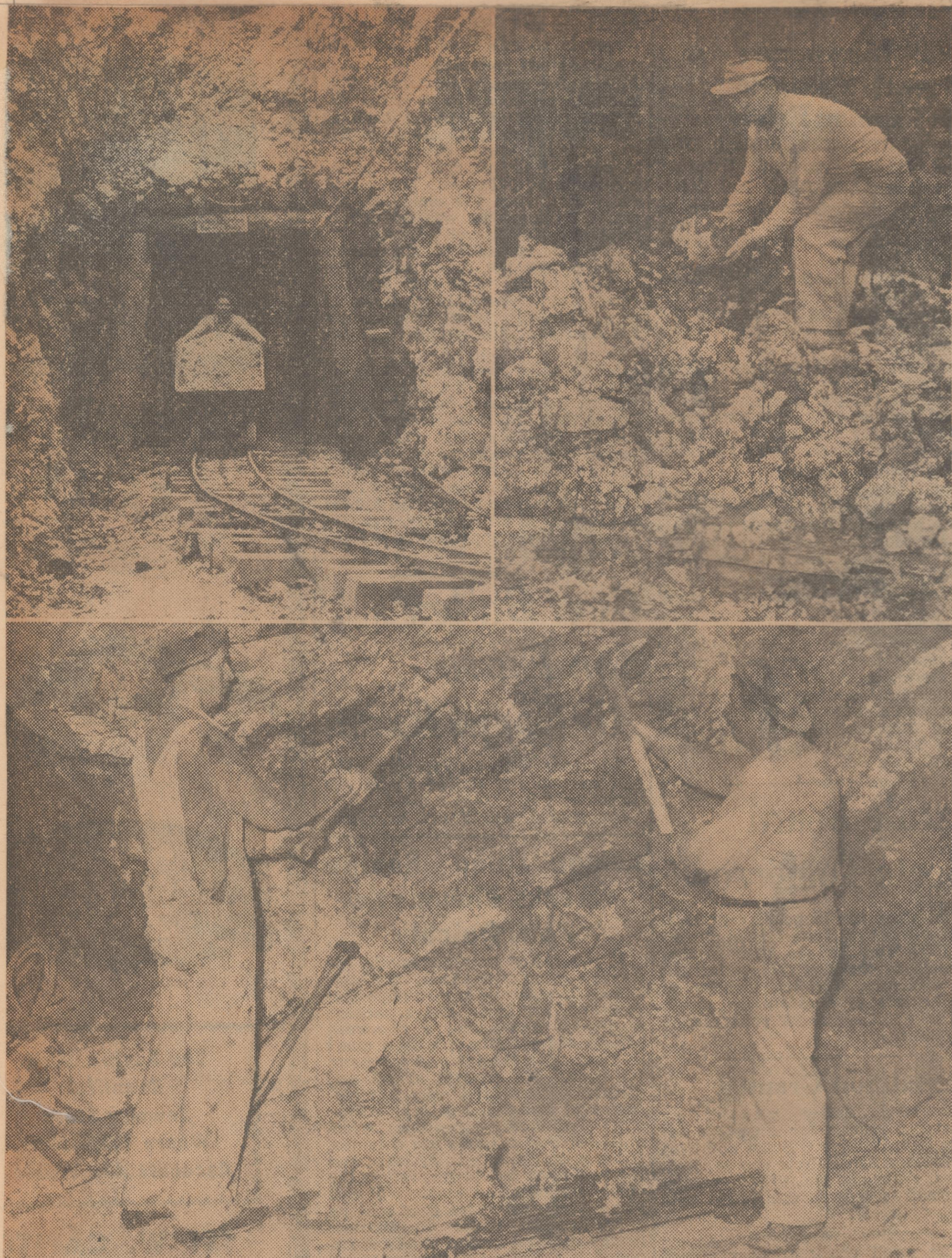
—Democrat Photo. Murfreesboro—From this mountainside, located deep in the Ouachita range, the North American Manganese Corporation plans to bring out thousands of tons of manganese ore for national defense purposes. In the top left picture a worker is shown riding out on a car of the ore. He is just emerging from a shaft, dynamited more than 350 feet straight back through the rock mountainside. Another shaft, and other planned shafts originating from the top of the mountain, will empty into the main shaft. There the cars will pick up the ore and bring it to the surface. In the top right picture a mine worker is displaying huge chunks of the ore, which is piled around the mine, stored there since its removal from the mountain as the shafts were being dug. In the bottom photo workers are pointing to a foot vein of the ore with their picks. (The ore is not broken out with picks, but dynamited out.)
