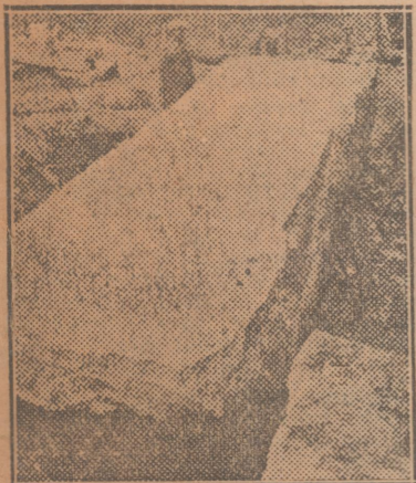
The block of pure marble pictured is one of the largest ever taken out of a quarry in the United States. It was quarried by the St. Claire Marble Company of Guion and contains 600 cubic feet. It is 24 feet long, 6 feet across, and 4 feet thick.
