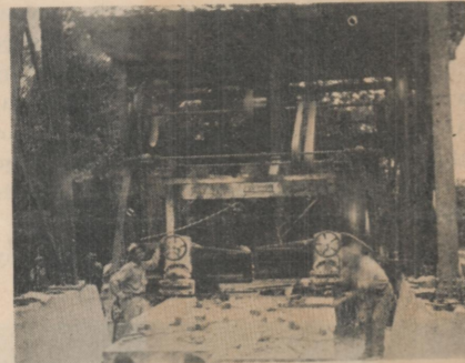
Surfacing Blocks With Stone Plane
