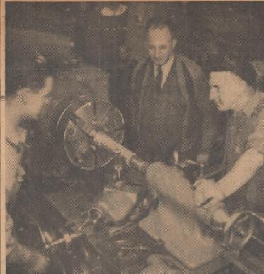
Adolph Chanosky, discoverer and developer of the new metal, chanite, which was named for him, is shown (center) in a laboratory of the United States Bureau of Mines at Salt Lake City. A piece of chanite has been welded to a steel drill. At the left is a piece of the hardest steel made. The chanite drill cut through it as though it were paper. The Bureau of Mines built a special furnace to process chanite, which has a
