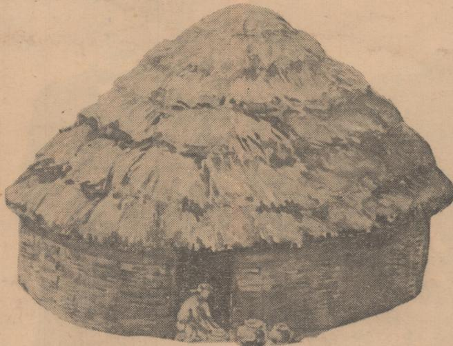
One of the cone-shaped houses of the Arkansas Caddo Indians made of reinforced mud with a thatched roof.
