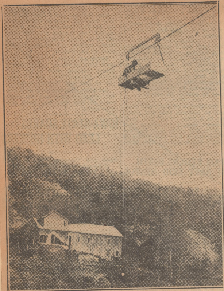
Methods of stream gauging for the utilization of water power in Arkansas are depicted in the photographs above. More than one-tenth of the available water power in Arkansas is now developed, or will be developed in the near future, according to Arkansas' stream gauging report No. 1, which has just been released by the Arkansas geological survey. At the left is shown how high water measurements are made from cable cars. This scene was made on the Buffalo river. At the right above is shown an engineer taking measurements by wading out into Mulberry river.
