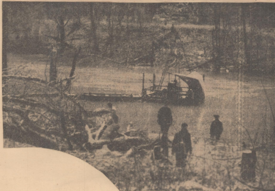
Core drilling in the middle of the Northfork river to test the dam foundation area is shown above.
